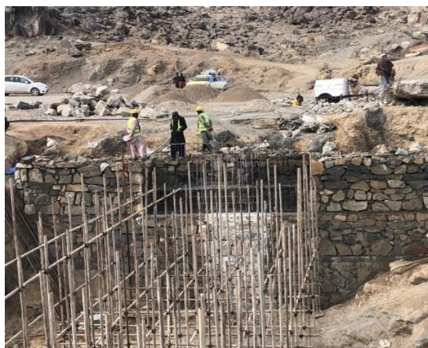
Photo 2 – Left: CfW participants remove the destroyed bridge, December 11, 2022. Photo 3 – Right: Reconstructing the foundation of Dahla Bridge, January 4, 2023.
